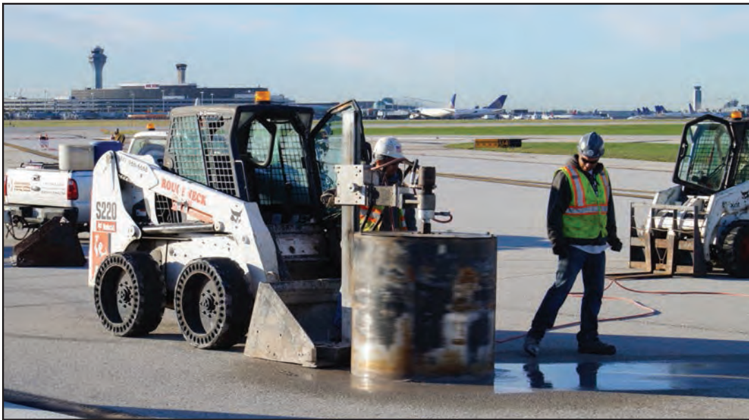
Figure 1. A 42 in. diameter core is used to extract the original runway light can.
