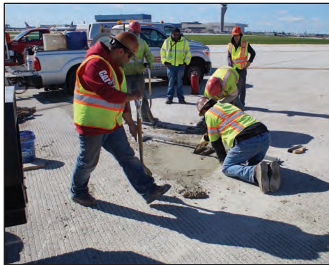
Figure 6. A rapid set topping mortar mix is used to finish the surface.
