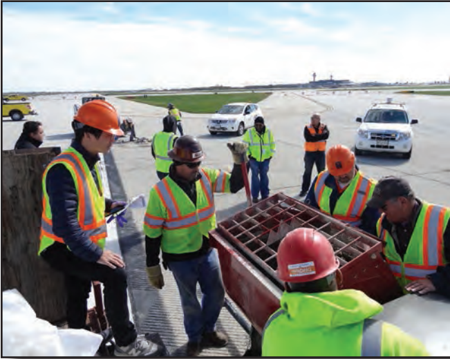
Figure 4. Grout is mixed on site using practical and field-appropriate methods.
