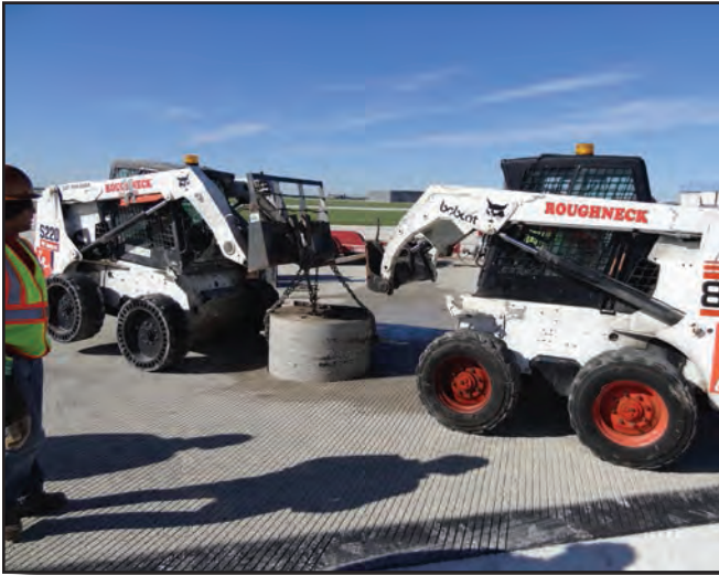
Figure 2. Lifting the core out of the pavement required clever teamwork.
