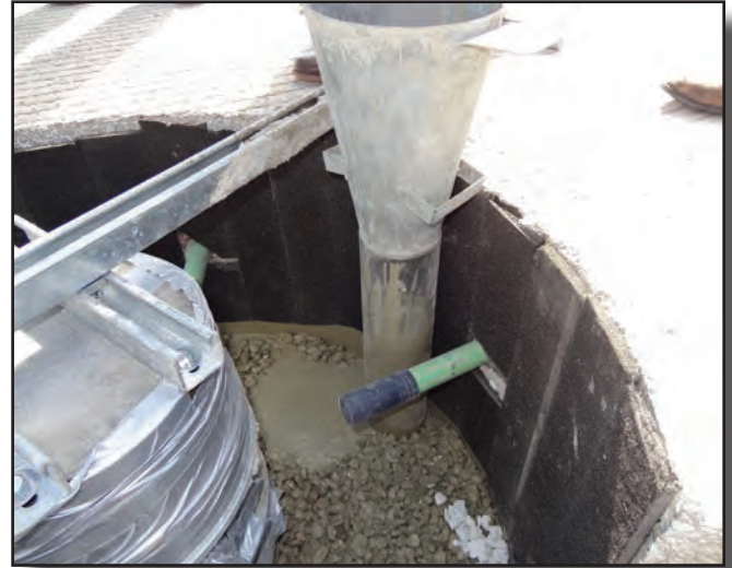
Figure 5. Grout is placed to saturate the pre-packed aggregate bed.
