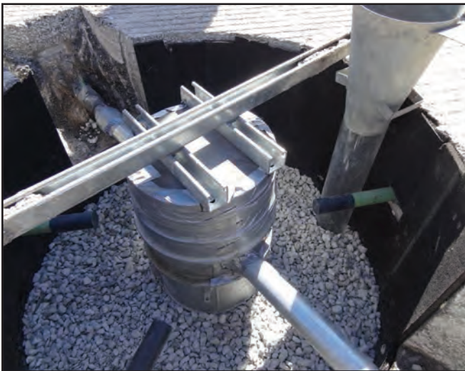
Figure 3. The new light can is installed with conduit for electrical connections.
