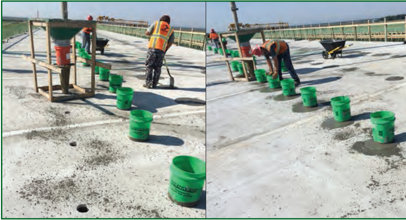
Figure 2. Placing SCC
