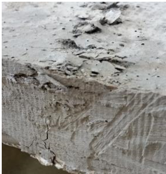
Figure 6.49. Tensile crack on panel SUC2
