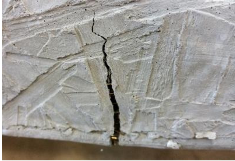
Figure 6.15. Tensile crack on panel FUW3
