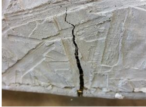
Figure 6.10. Tensile crack on panel FUC3
