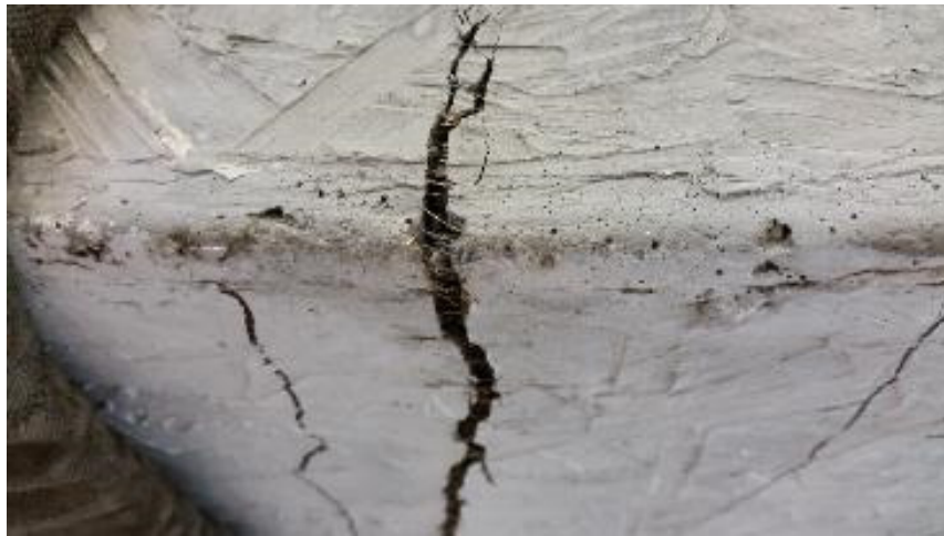
Figure 6.44. Tensile crack on panel SUN3
