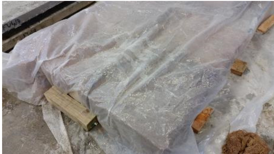
Figure 5.11. Plastic sheet on top of burlap
