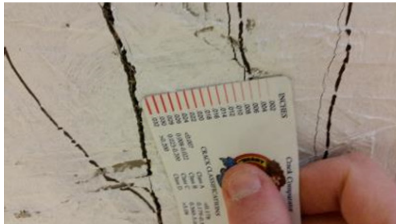
Figure 6.28. Crack widths of panel FUN2
