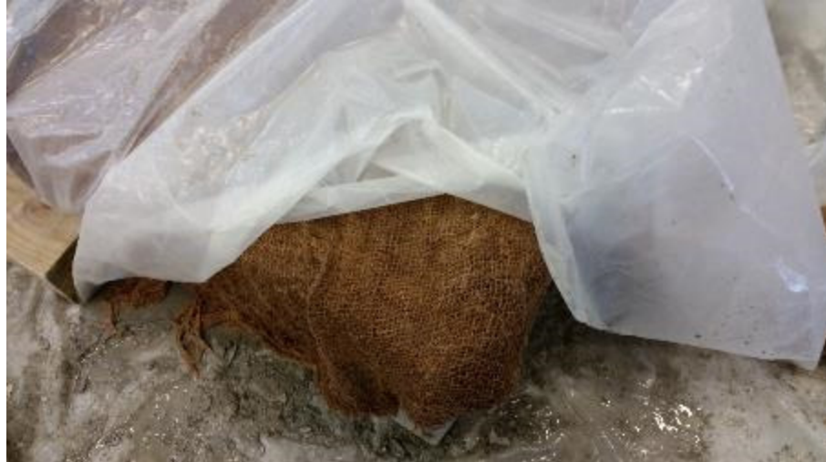
Figure 5.10. Wet burlap on top of concrete surface
