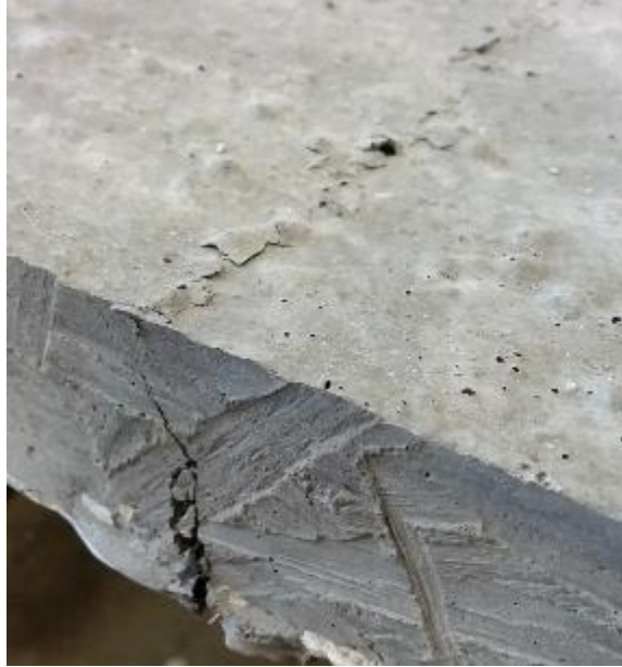
Figure 6.55. Tensile crack on panel SUN2
