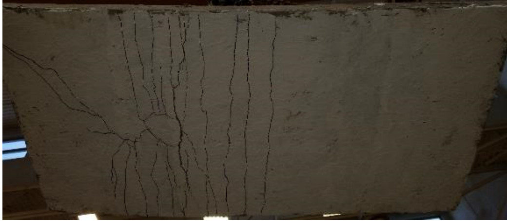
Figure 6.50. Crack pattern formation at the tension face of panel SUC2
