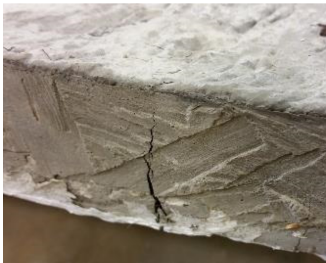
Figure 6.26. Tensile crack on panel FUN2
