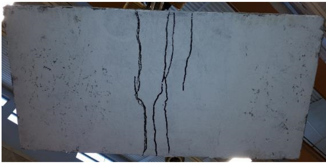
Figure 6.20. Crack pattern formation at the tension face of panel FUN3
