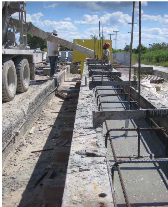
Figure 34. Casting of concrete beam from one side.
