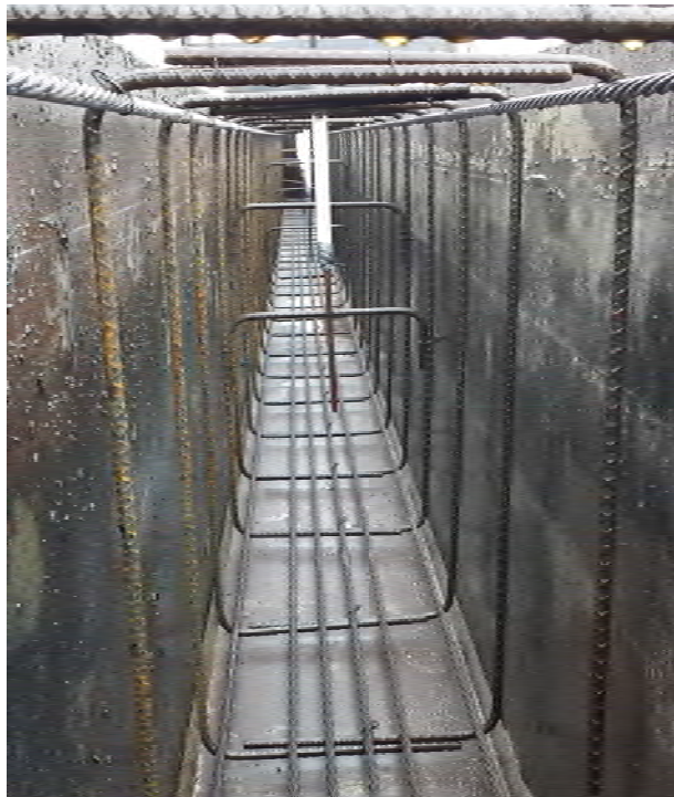
Figure 32. Reinforcement configuration in rectangular beams.
