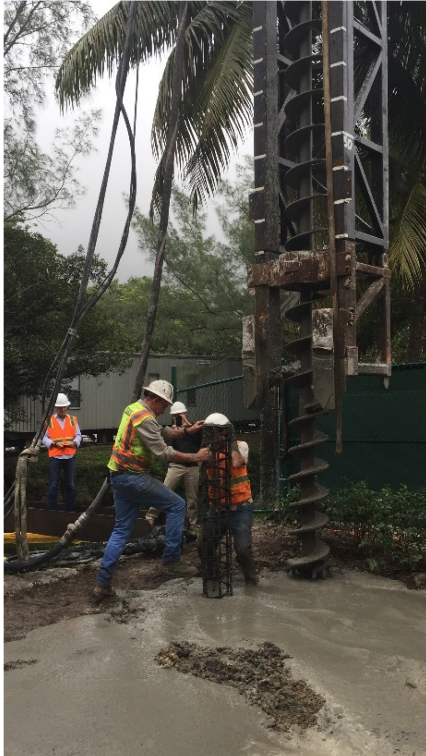
Figure 6: Construction of auger-cast pile
