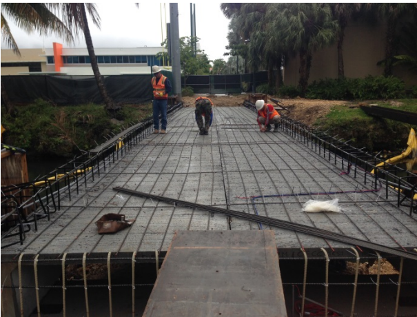
File cap preparation, girder setup, and deck instrumentation and construction
