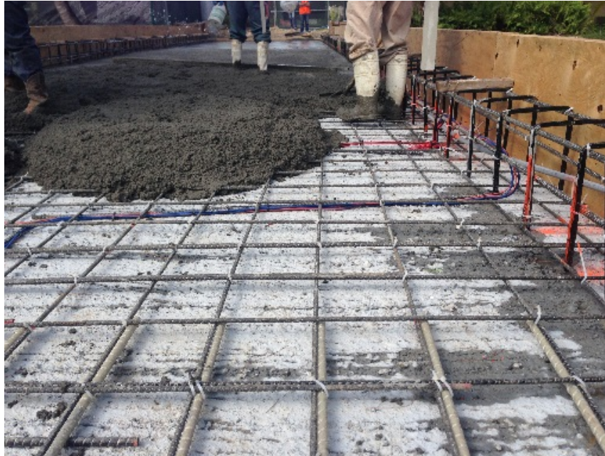
Figure 10: Casting of the deck topping
