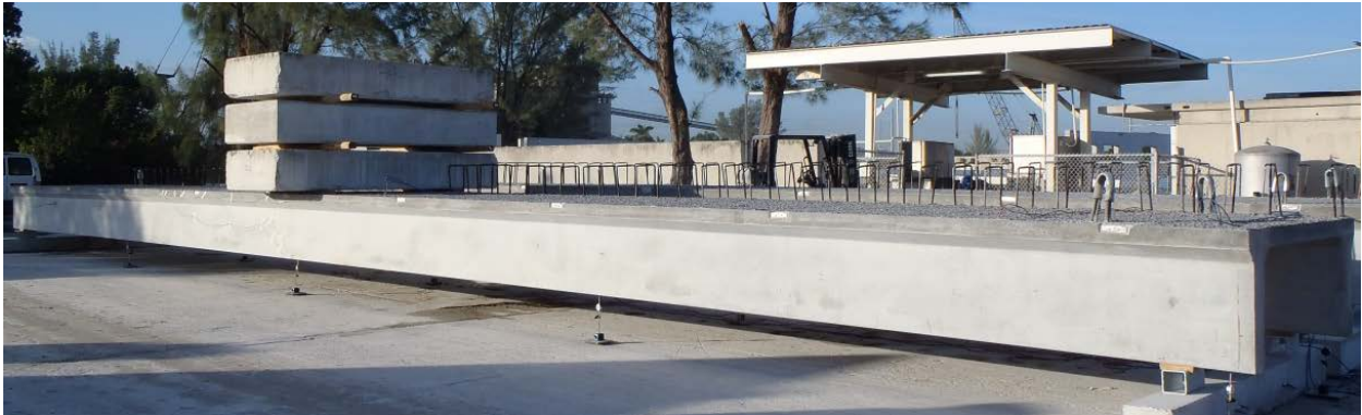
Figure 8: DT girder loaded under a three-point-load setup
