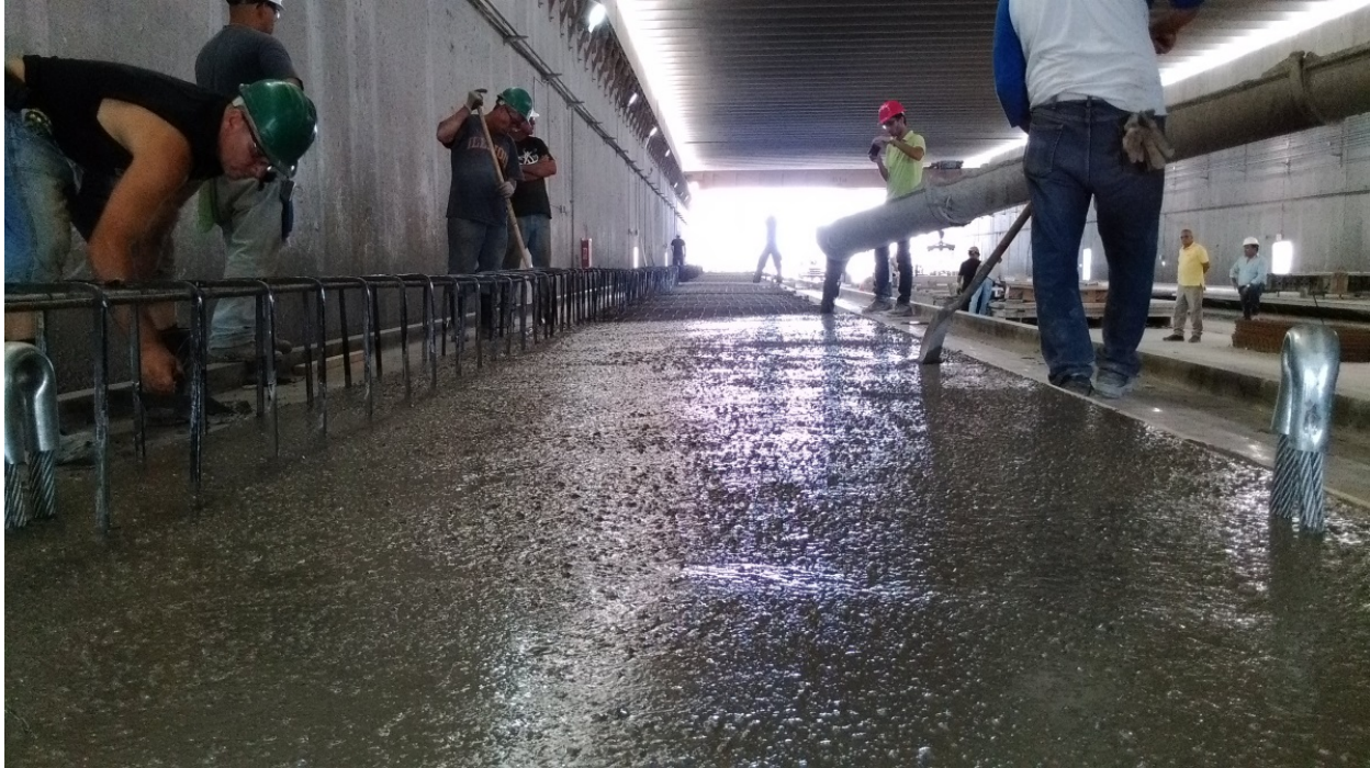
Figure 5: Concrete pouring phase
