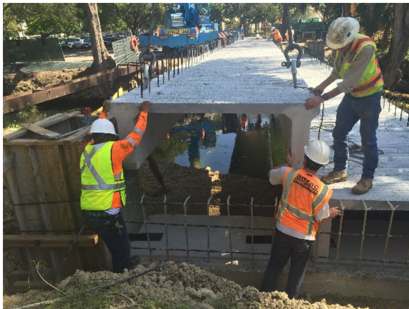
Figure 9: Installation of girder
