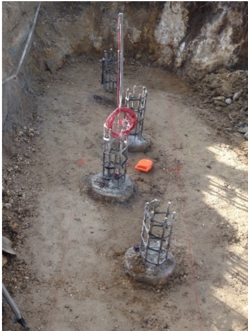
Figure 7: Exposed reinforcement in piles
