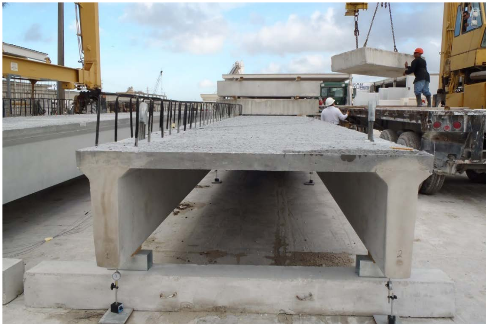
Figure 9: DT girder loading phase, dial gauges and supports
