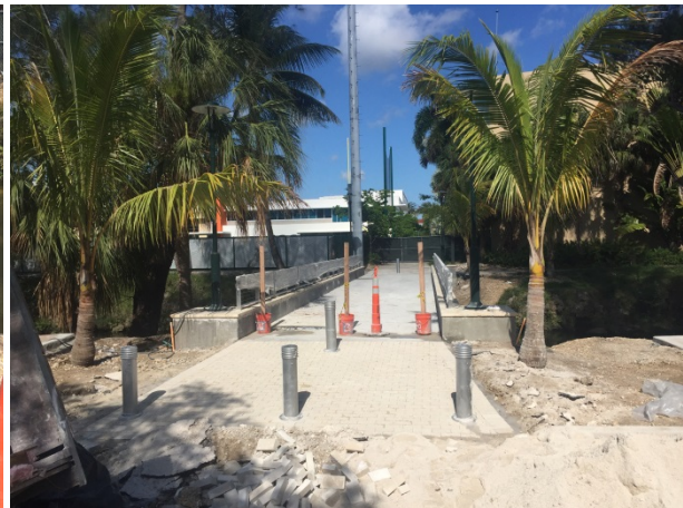
Deck and curbs casting, and railing installation
