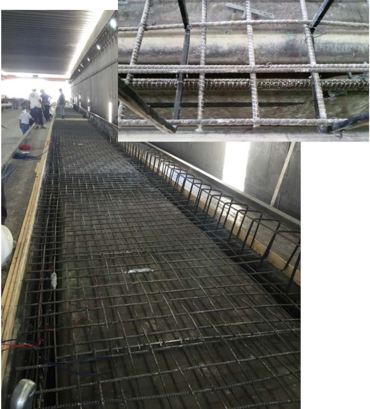
Figure 2: Double-tees casting bed and detail of BFRP reinforcement at casting
