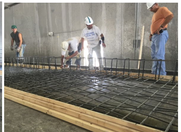
PC girder instrumentation and construction
