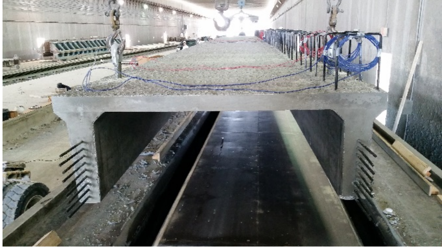
Figure 3: Double-tee being lifted from the casting bed
