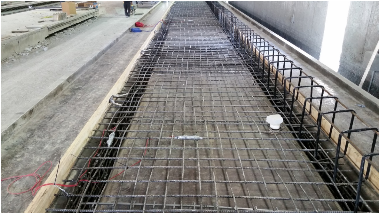
Figure 3: BFRP reinforcement and CFRP tendons arranged in the Coreslab prestressing bed
