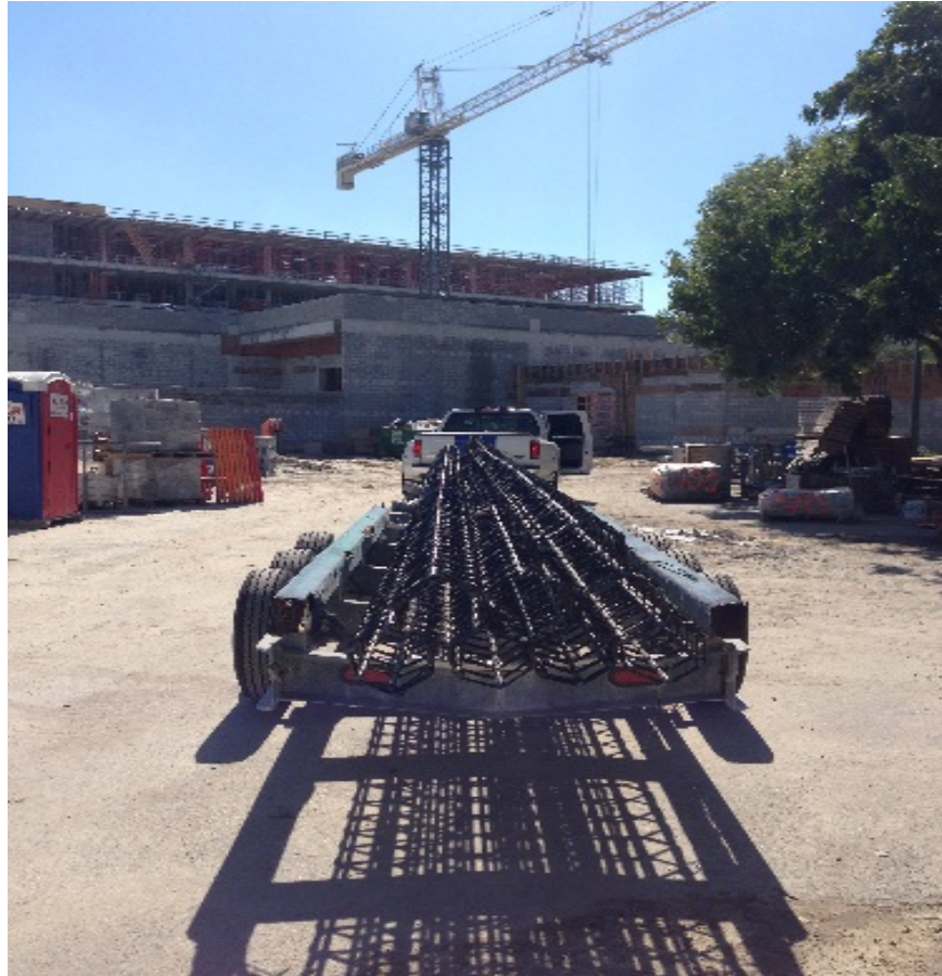
Figure 5: Delivery of BFRP pile cages at the site
