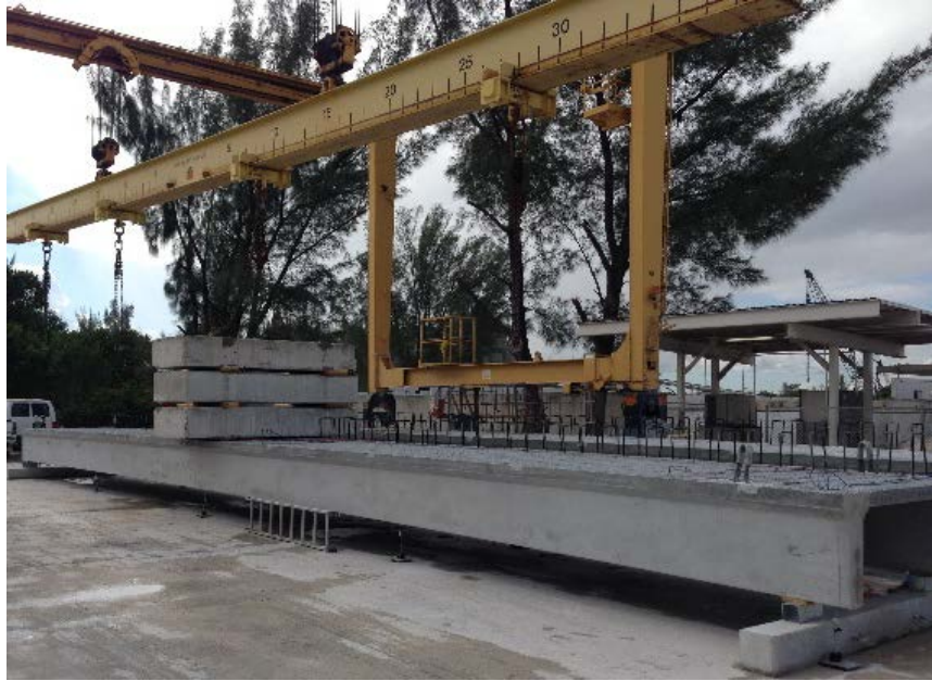
Figure 11: Double-tee static load test at precast yard
