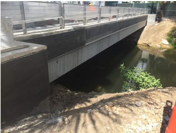
Deck and curbs casting, and railing installation
