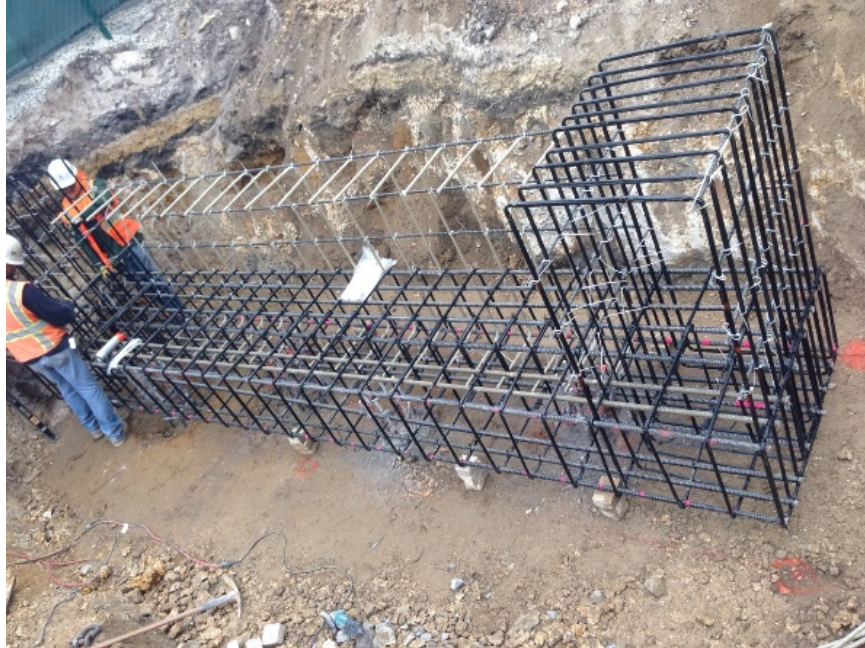
Figure 8: Reinforcement cage for pile cap, side blocks and back-wall
