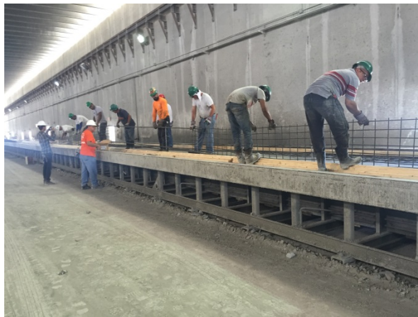
PC girder instrumentation and construction
