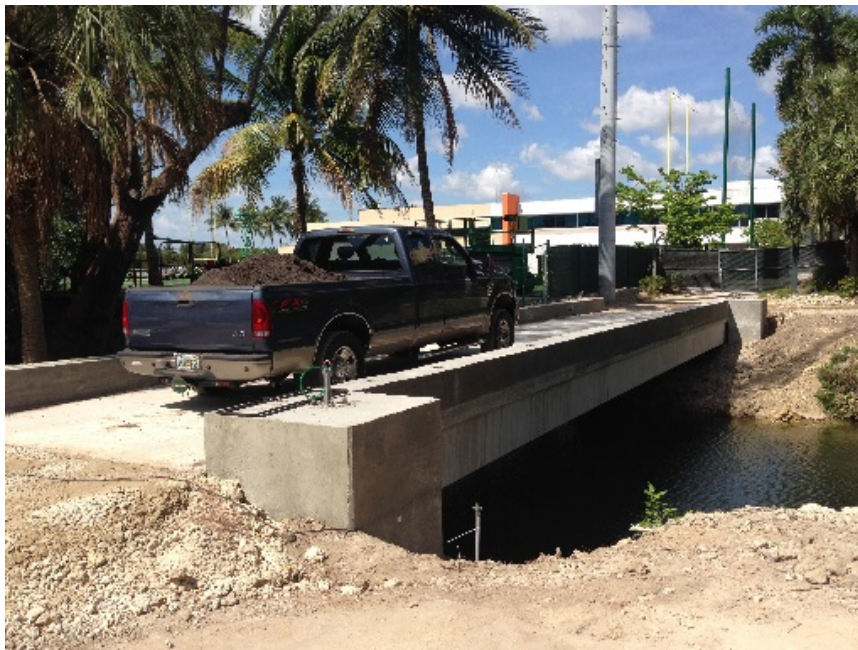
Figure 12: Load test at completion of superstructure construction
