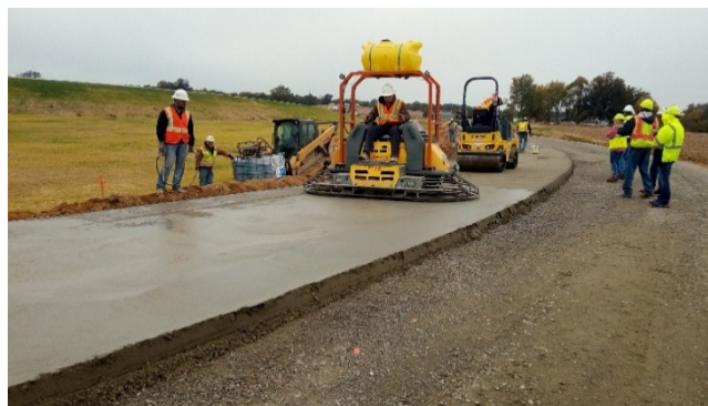
Figure 12 - Finishing process
