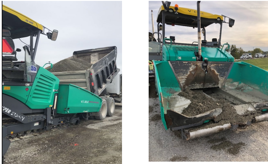
Figure 10 - Loading process of the slip-form paving
