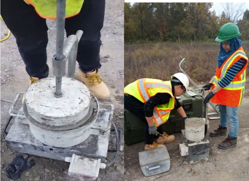
Figure 15 – Vebe test apparatus for determining consistency/density of fresh CCP
