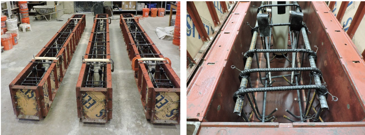
Figure 5.8: Upside Down Placement of Cages (l) and Protection of Exposed Portion of Stirrups (r)
