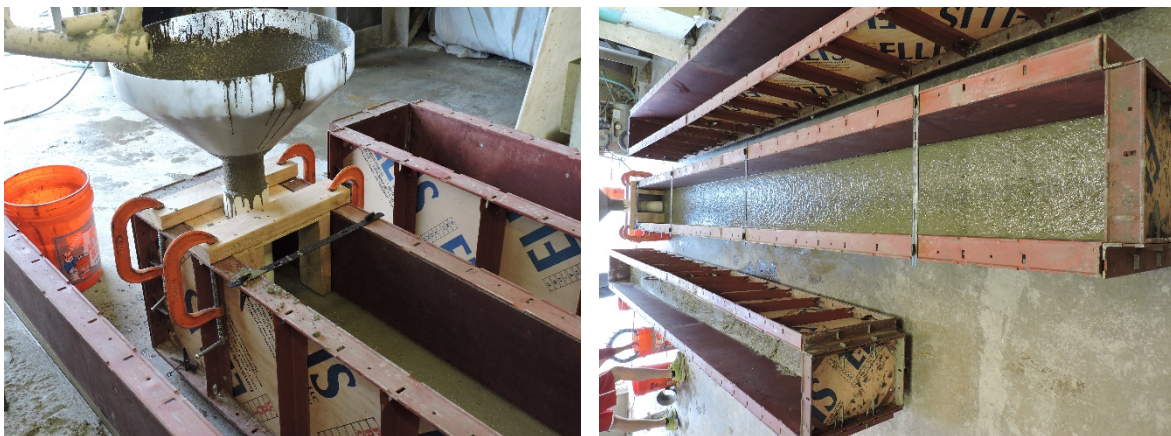
Figure 3.2: Full-Scale Flow Test of FR-SCC Mix Design, 15% Type K Expansive Agent
