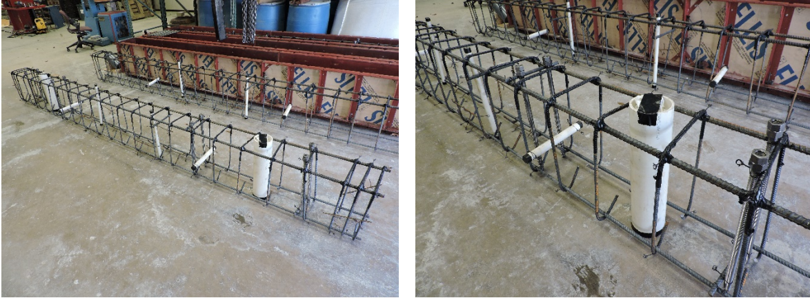
Figure 5.7: Reinforcing Cages with PVC Inserts for Access Ports, Vent Holes, and Pick Points
