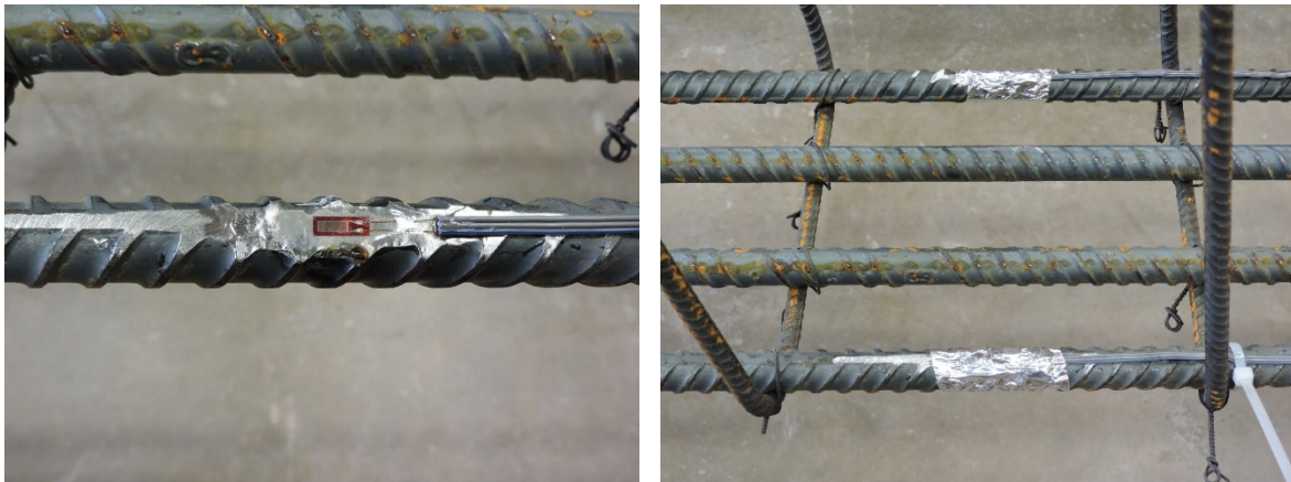
Figure 5.3: Strain Gages Installed Near Midspan of Longitudinal Reinforcing Steel
