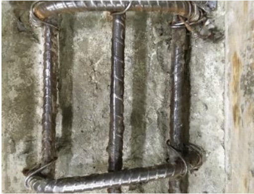
(a) Cleaned reinforcement before repair
