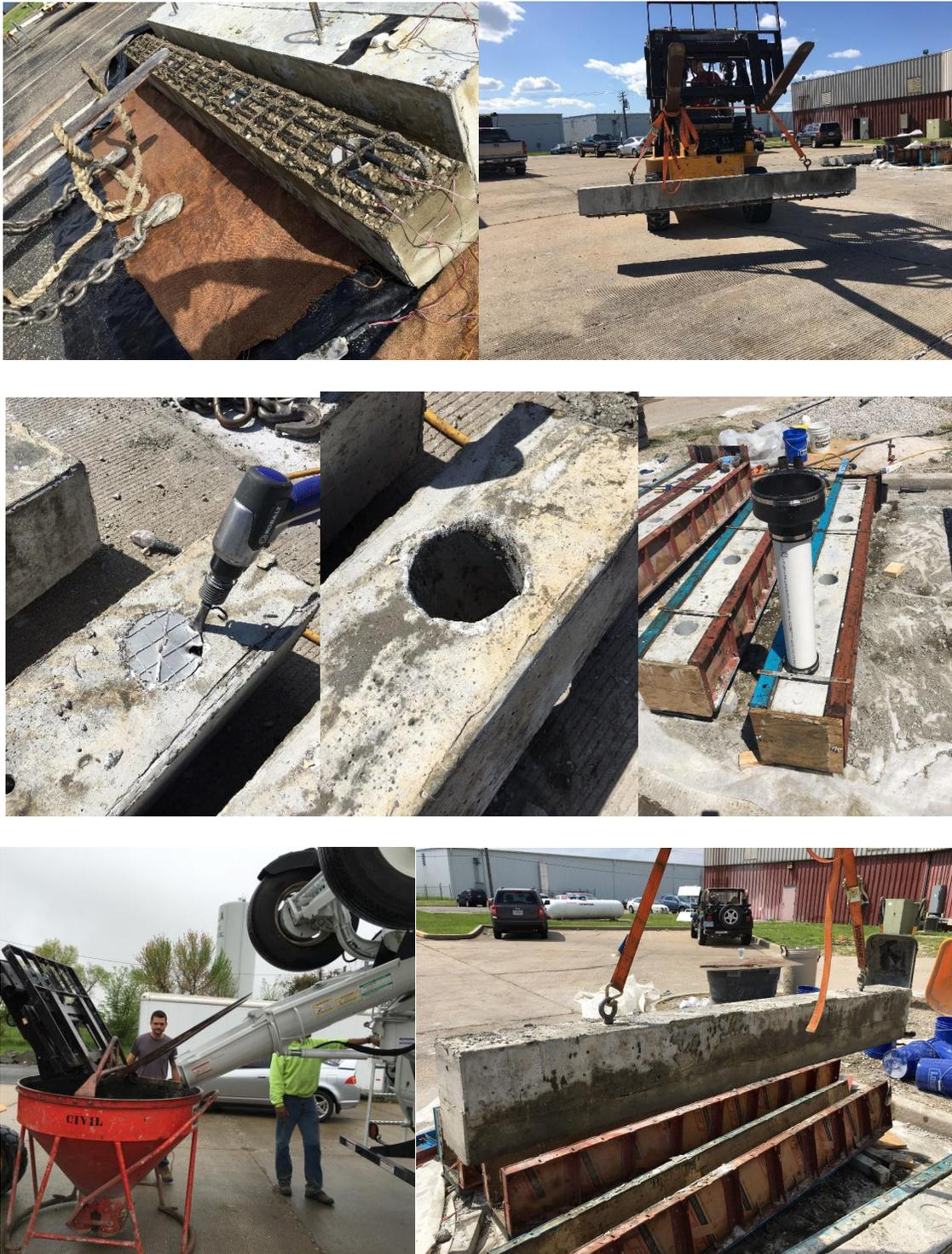
**Figure 5-11: Repairing of CVC Beams using FR-SCC**
