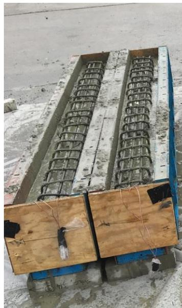
**Figure 5-9: Substrate casting (of the 2/3 upper beam height) in inverted position**
