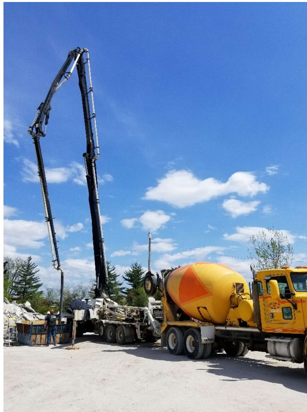
Figure 59. Pumping boom in A-shape configuration.
