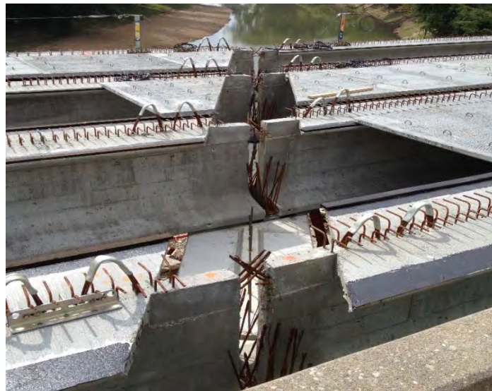
Figure 2.12 Highway-50 bridge intermediate bent with MoDOT end girder detail
