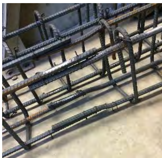
Figure 3.4 Straight-lap detail
