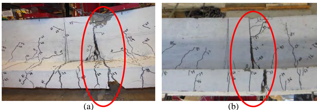
Figure 6.24 Failure mode (a) B-4-U-MB-M (b) B-5-U-U-M
