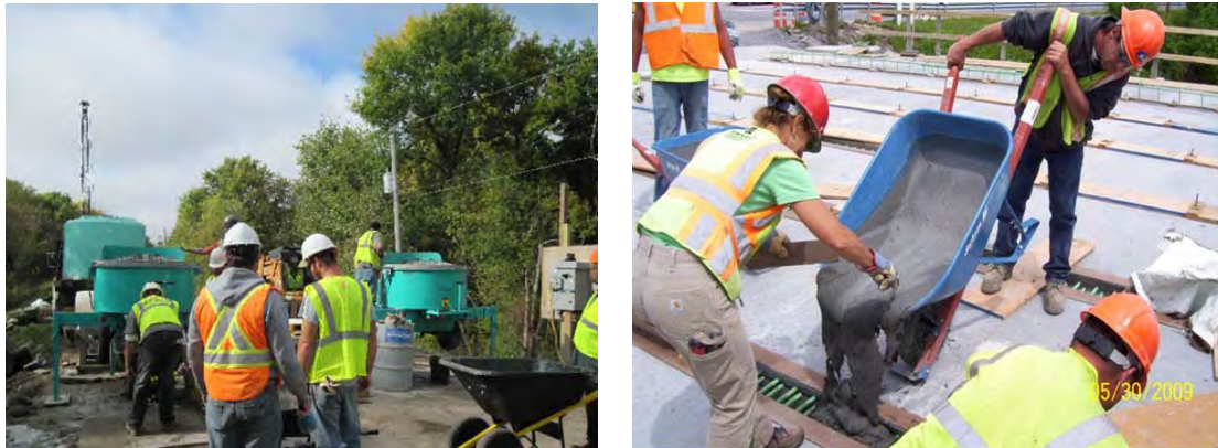
Figure 2.2 Batching and casting UHPC at site (FHWA, 2016)
