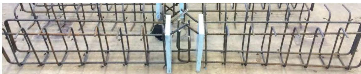
Figure 3.9 Reinforcement layout with joint detail
