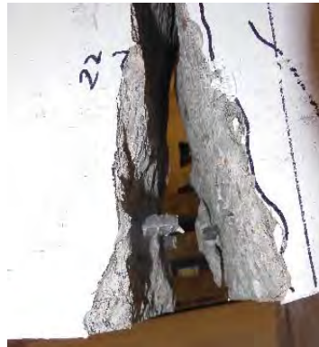
(d) Specimen B-21-U-S-H showing rebar rupture Figure 6.18 UHSC hairpin specimens at failure
