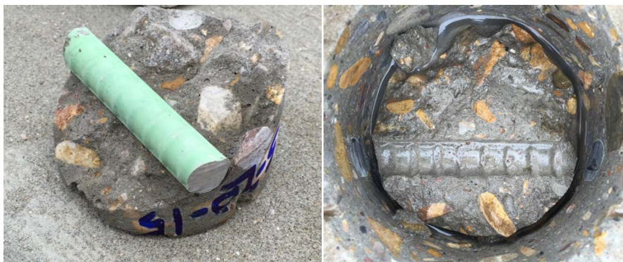
Extracted epoxy-coated steel rebar sent to OC (left) and its footprint (right)
