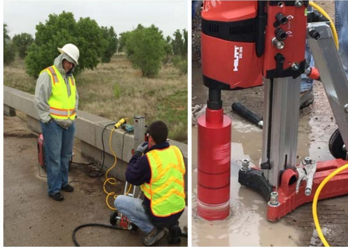
Figure 4: Concrete core extraction from the bridge deck
