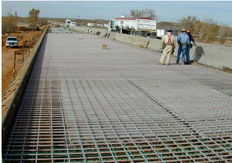
Bottom mat epoxy coated steel rebars [5]
