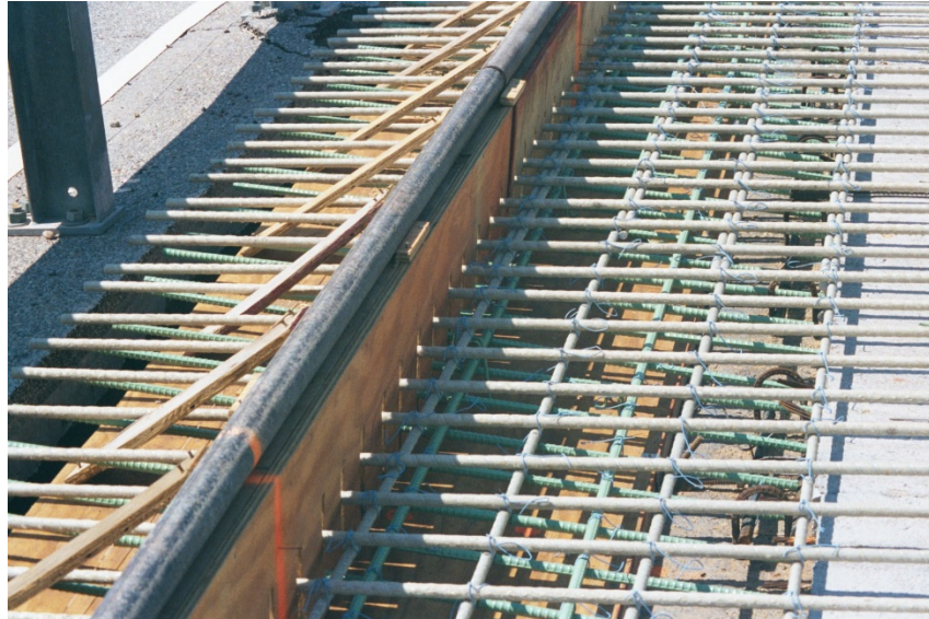
GFRP bars in slab overhang adjacent to phased construction [8]
