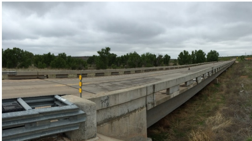
Figure 1: Sierrita de la Cruz Creek Bridge, Amarillo, Texas
