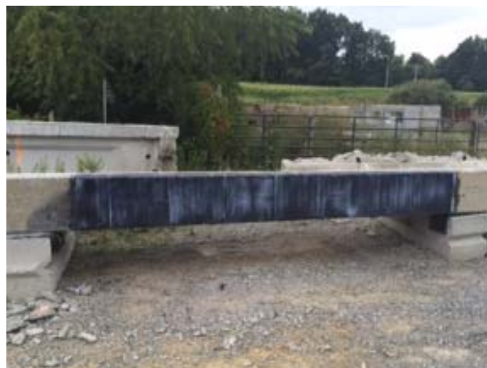
Figure 4-23 – FRP Strengthened Girder
