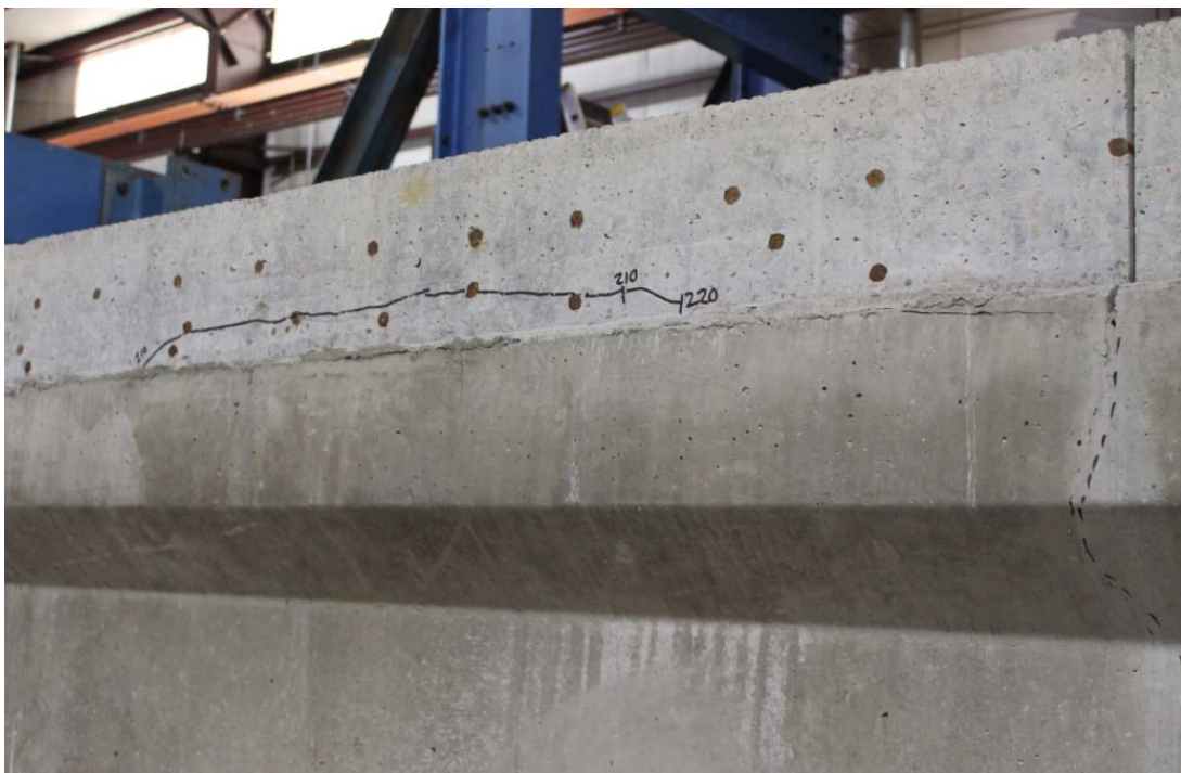
Figure 4-36 – Test 5 – Horizontal Shear Cracking and Crack Propagation at Gap
