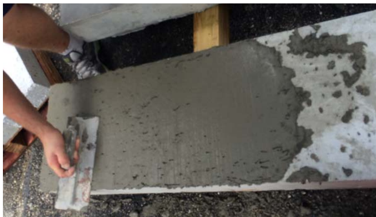
Figure 2-17 – Repair Mortar Application
