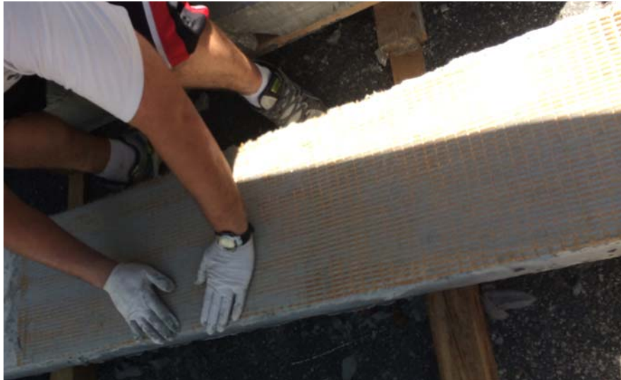
Figure 2-18 – FRCM Application Over Repair Mortar
