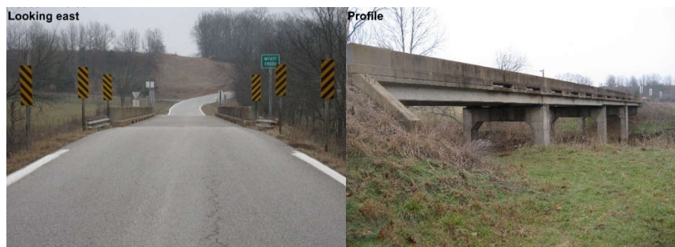
Figure 3-2. Bridge P-0058 Approach and Profile View
