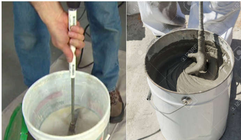
Figure 4-4. Mixing Resin and Cementitious Matrix
