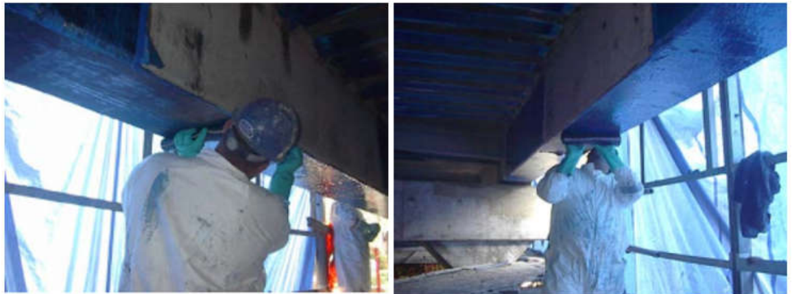
Figure 4-6. Manual Layup of CFRP
