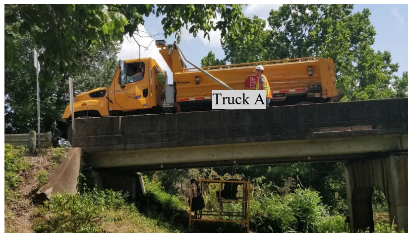
Figure 5-8. Truck on Span 4 for Load Test
