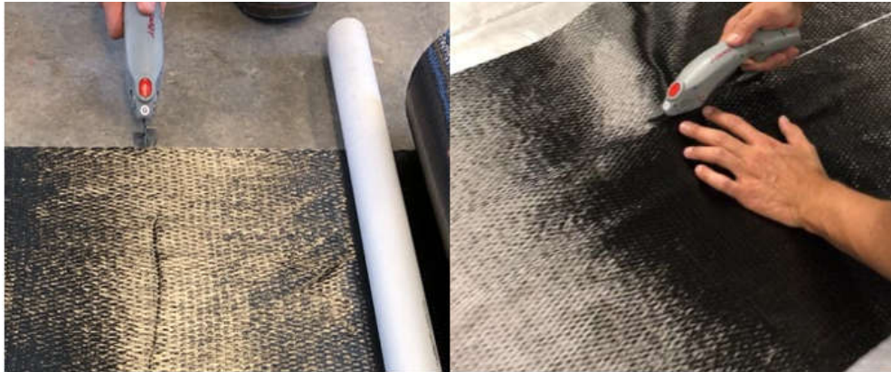
Figure 4-5. Preparation of CFRP Sheets
